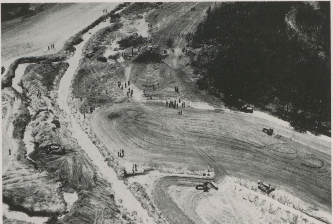
A new channel is dug for Reinhardt Creek.
