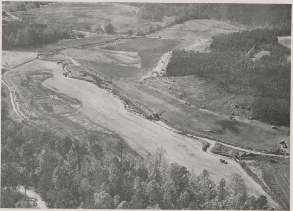
Aerial view of drag-line shovel at work.
