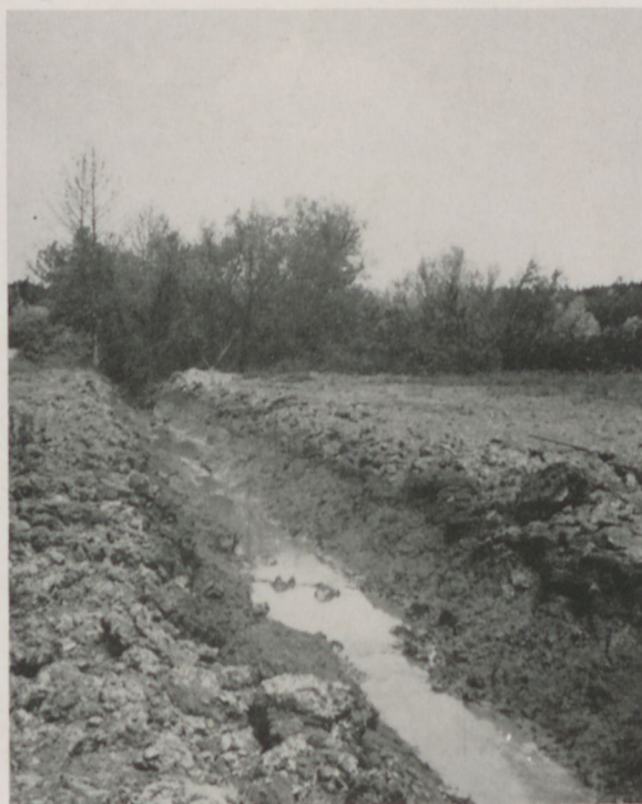
4,000 feet of ditches dynamited.
