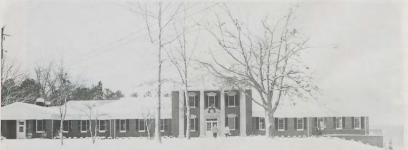
The finished product under a foot of snow.
