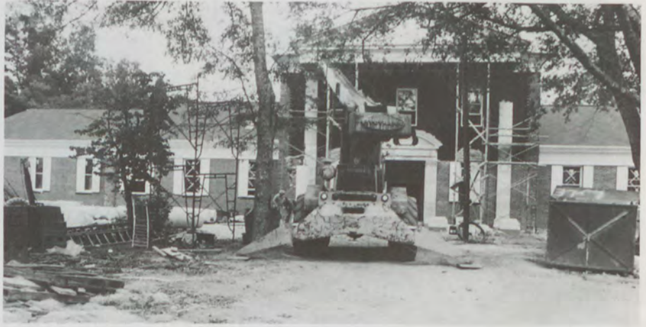
The Gordy Center under construction.
