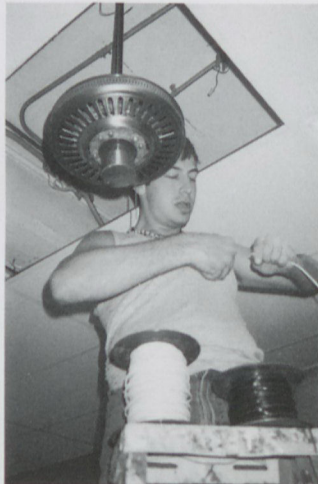
Troy Hamilton installs a ceiling fan in the kitchen at Red Bird Mission.
